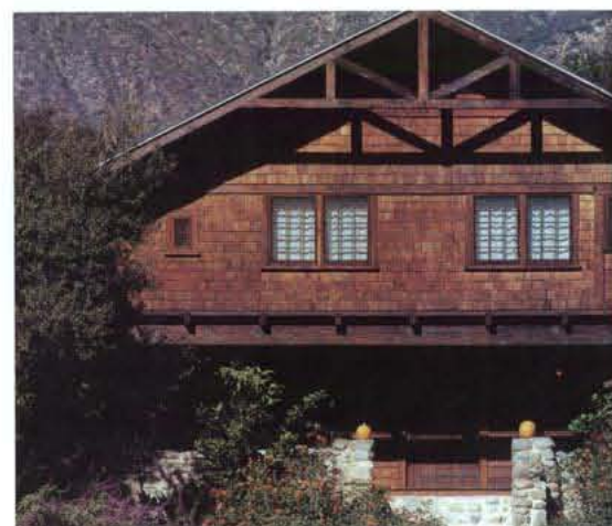
TIMBER TRUSS & WOOD SIDING
