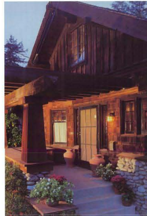
MAIN ENTRY WITH TIMBER TRESTLE
